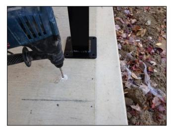
**Step 5:** Bolt down posts using the correct type of fastener (not provided) needed for the surface you are mounting to.
