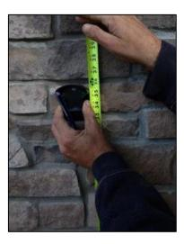
**Step 4:** Mark and Pre-Drill holes for post attachment.
