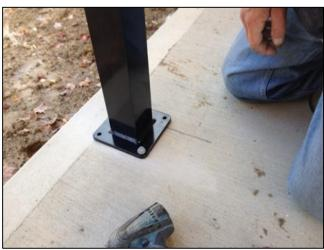
**Step 6:** Slide brackets onto horizontal rails of the section and attach to posts using the stainless steel self-tapping screws provided if hanging the section onto aluminum posts. If attaching to existing wood posts or brick wall, use the correct type of fastener (not provided) needed.
