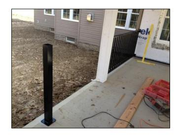
**Step 3:** Measure and mark locations where brackets will be hung on either the aluminum posts or on existing posts or walls.
